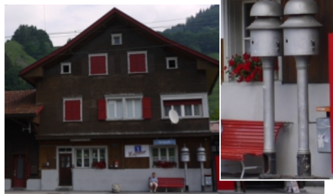
The stations of Cavadürli (above) and Grüşch (down) have / had a signal bell with ground wirel.
